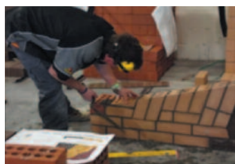
Ben Roche Bricklaying
